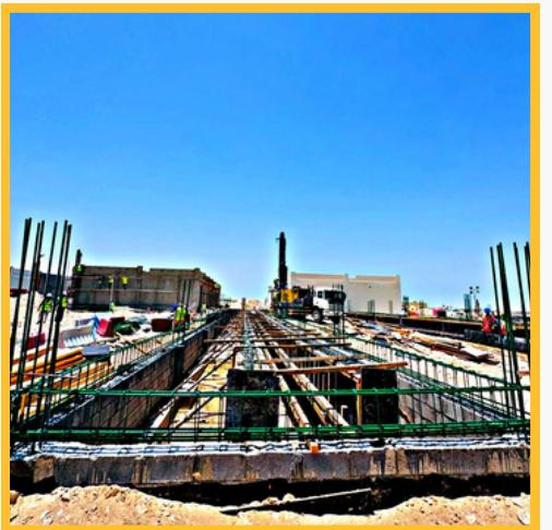
**Scope :** Execution of steel fixing and block work for structural
